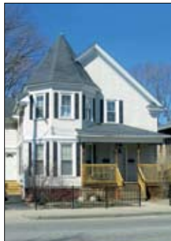
Jefferson Boulevard, Warwick Family apartments developed by the House of Hope Community Development Corporation
